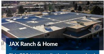
This 320 kW installation is comprised of 867 modules and 4 string inverters. The solar system is expected to cover 100% of their energy usage and produce 472.2 MWh annually.
