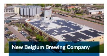
Namasté Solar installed the 300 kW rooftop system on their bottling plant's 25,000 square-foot rooftop. The system provides up to 13% of the plant's electricity needs.
